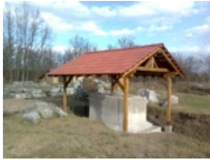
Figure 5 (upper left): new roof over statue base, Nicopolis ad Istrum.
